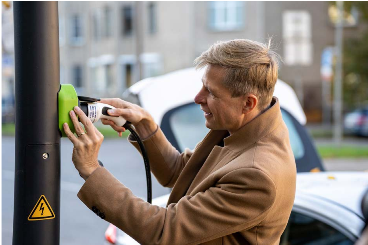
Picture 7. 1 Street lighting poles with electric car charging station.
