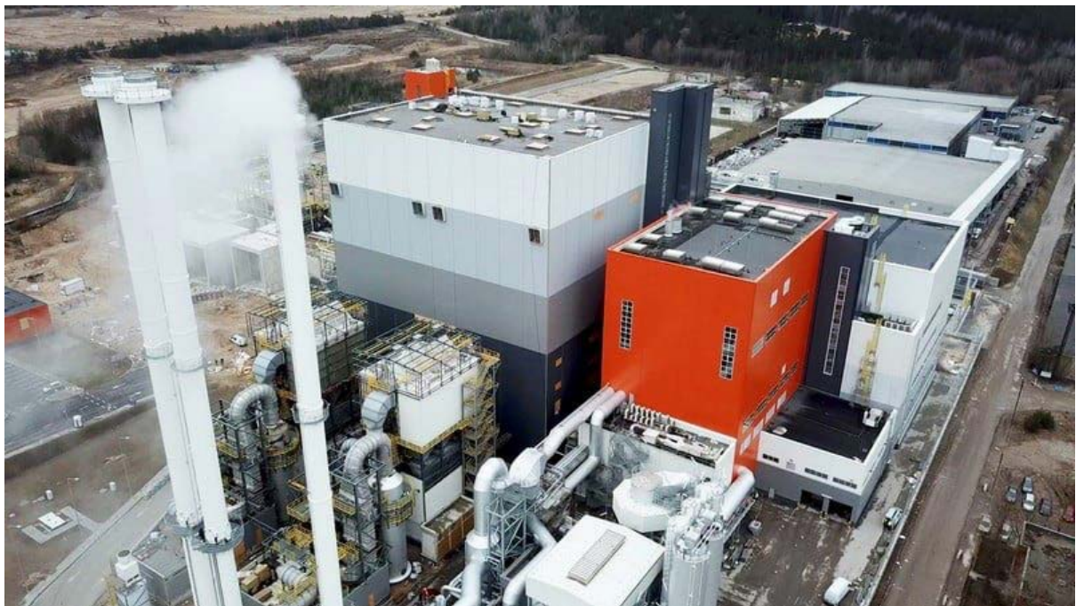
Picture 7. 10 Vilnius biofuel cogeneration facilities will be fully functioning in 2024.
